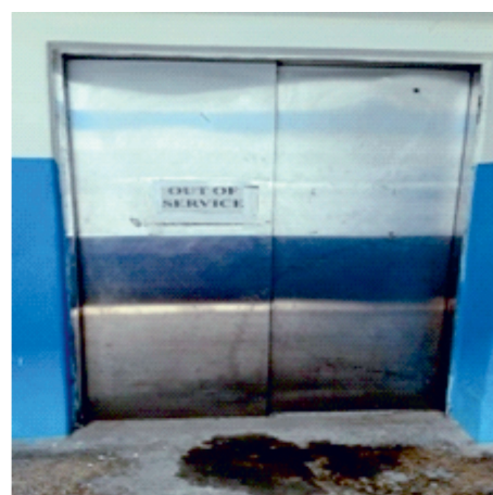
Out-of-order lift at Aizawl CH
